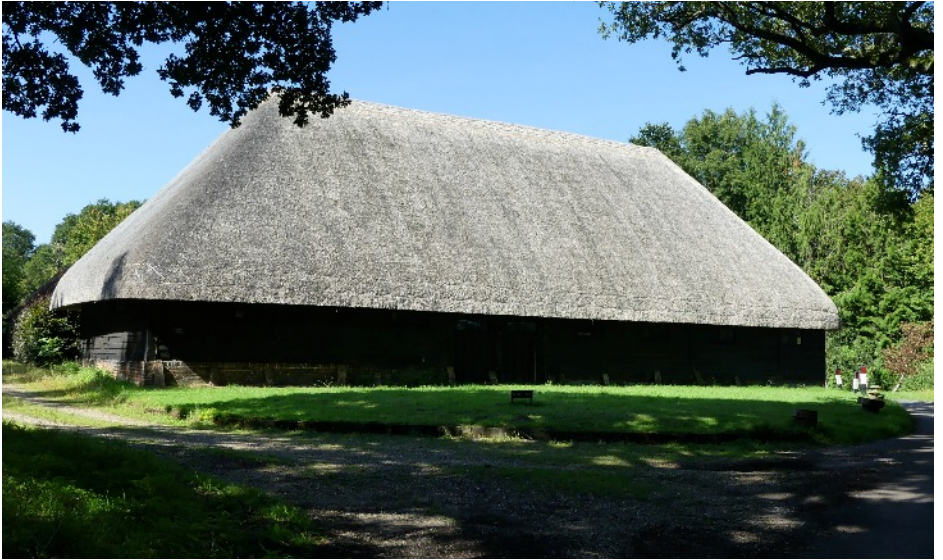
The great barn at Tadley Place looking superb with its newly thatched roof.
