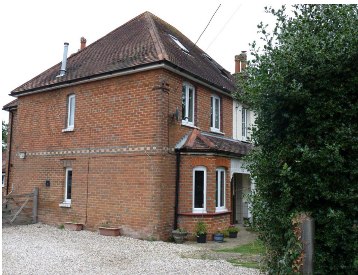
Eliza Wells house was 'Arundel Cottage', Franklin Avenue, Tadley. It is located to the west of the Holmwood Healthcentre.
